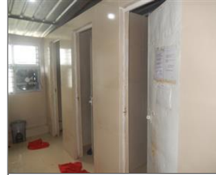
Photo of the sanitary facilities Toilet.JPG
