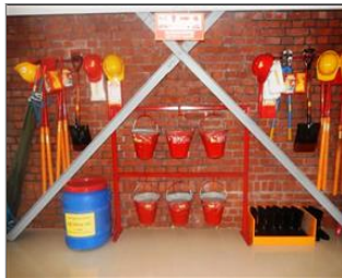
Photo of the inside of the main production hall Firefighting equipments.JPG
